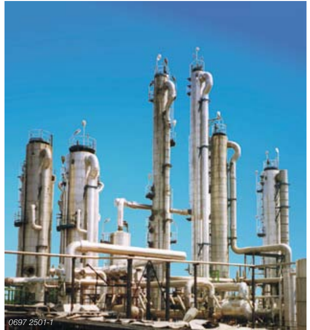
DMAc recovery plant
